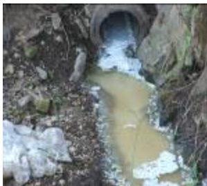
Wash water off parking lot
